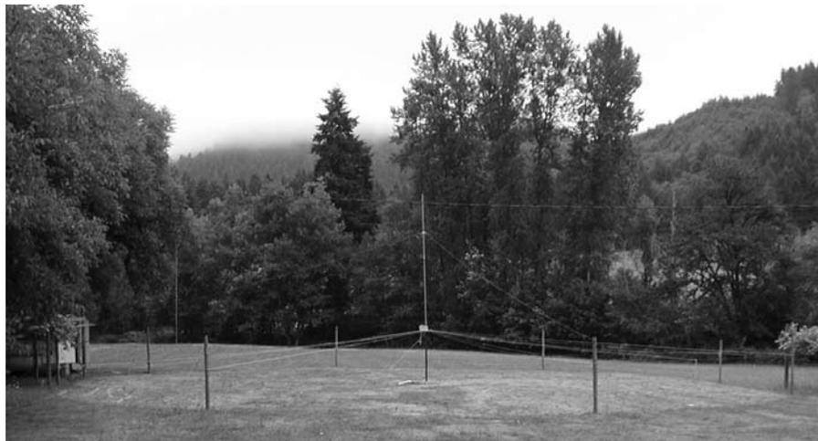
Figure 1 — Here is a view of the vertical with elevated radials.
